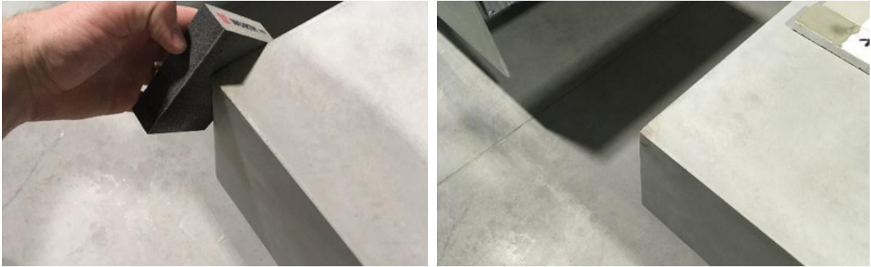
Photo: Example of additional sanding of the repaired area and its final appearance
