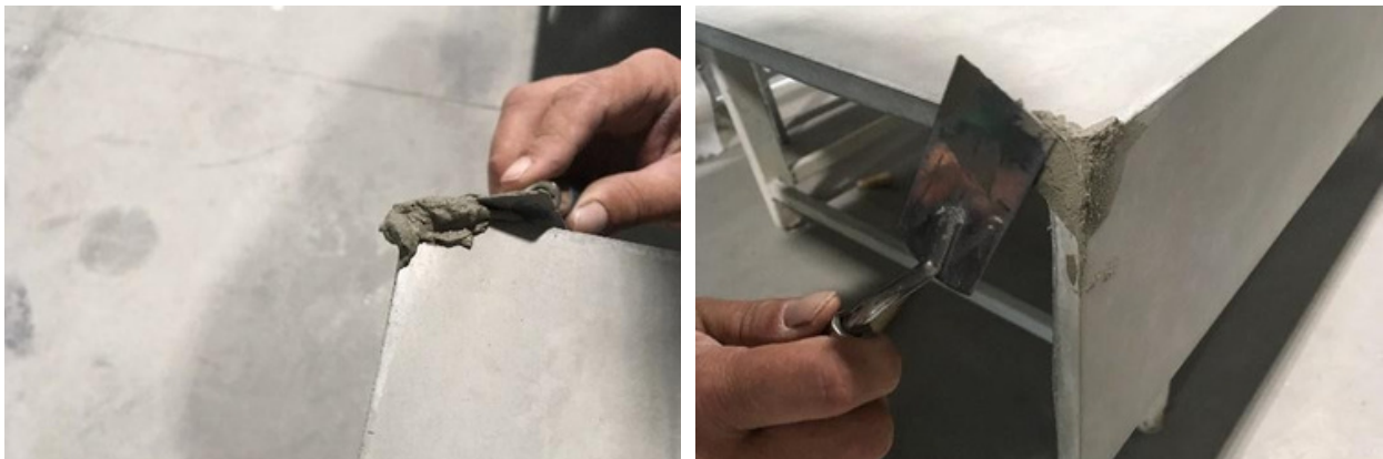
Photo: Examples of application of the repair compound
